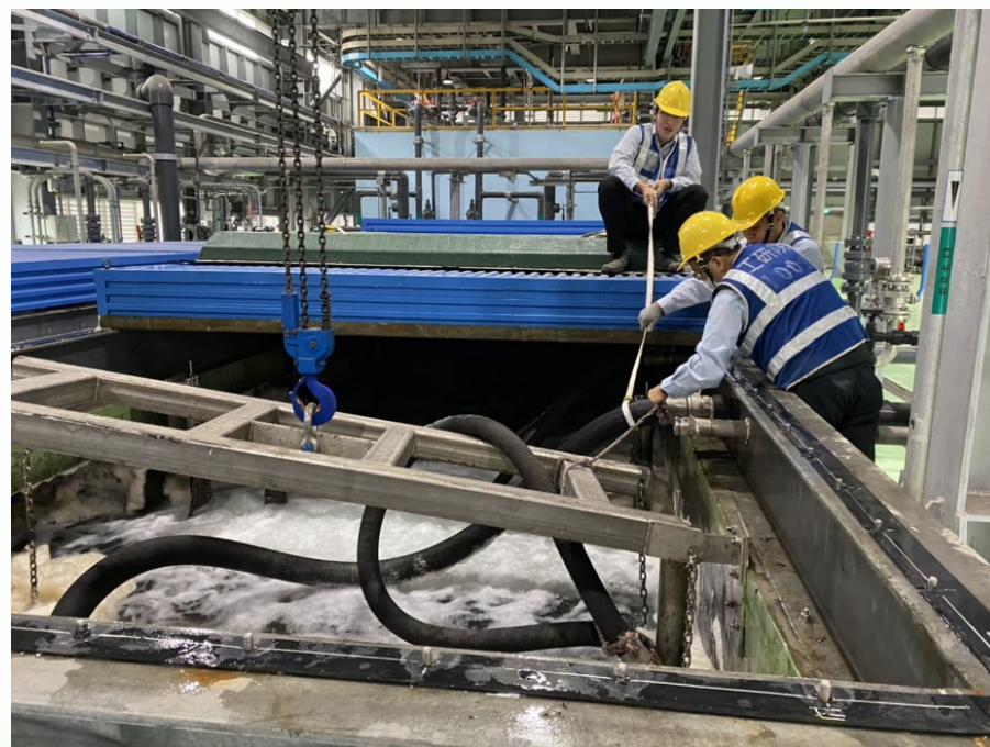
SMF rack lifting operation
