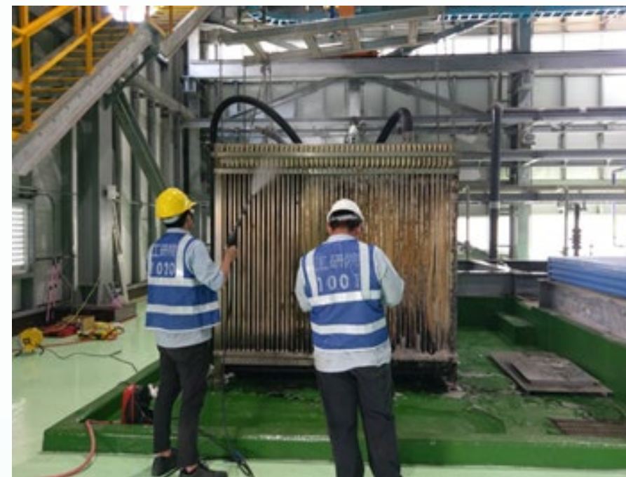
Spray the membrane with a hose to remove surface contamination
