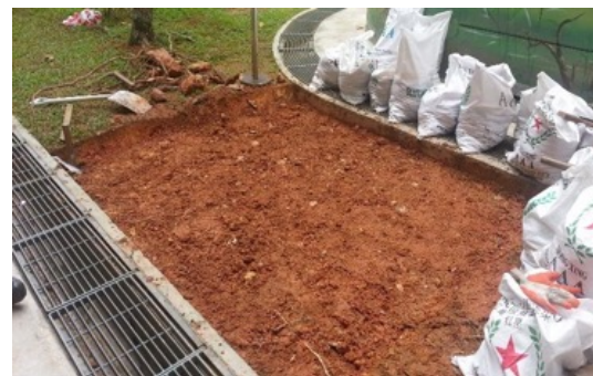
Bioretention site filled with engineered soil 1
