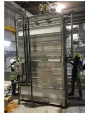
Full-scale flat sheet ceramic membrane at Changi WRP
