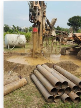
Anti-drought well at Taichung Central Park Drilling work
