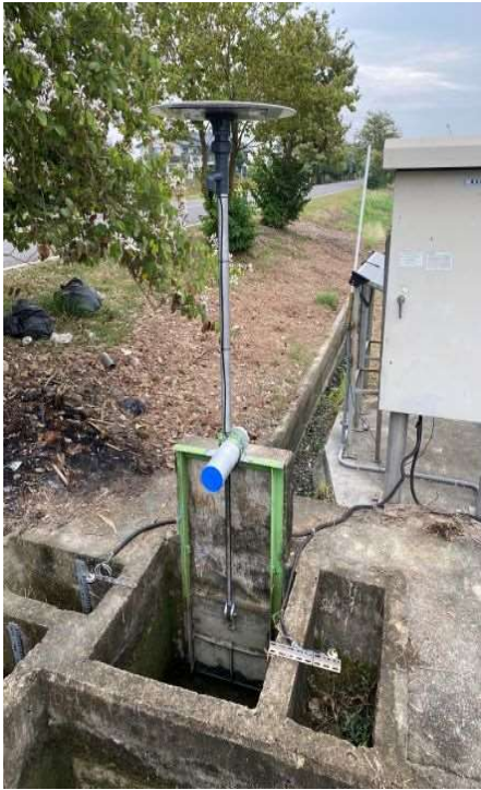
Watergate(Electric) ,(TSMC)
